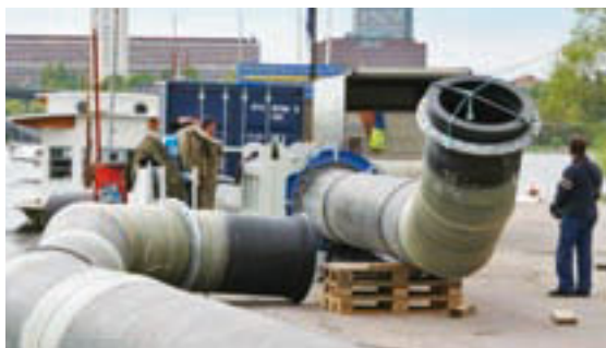
FOTO: FROG CONSTRUCTION & DIVING
